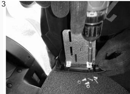
3 Put the mounting brackets on the new fascia plate provided and fix them with screws. Pay attention to the letters on the brackets.
